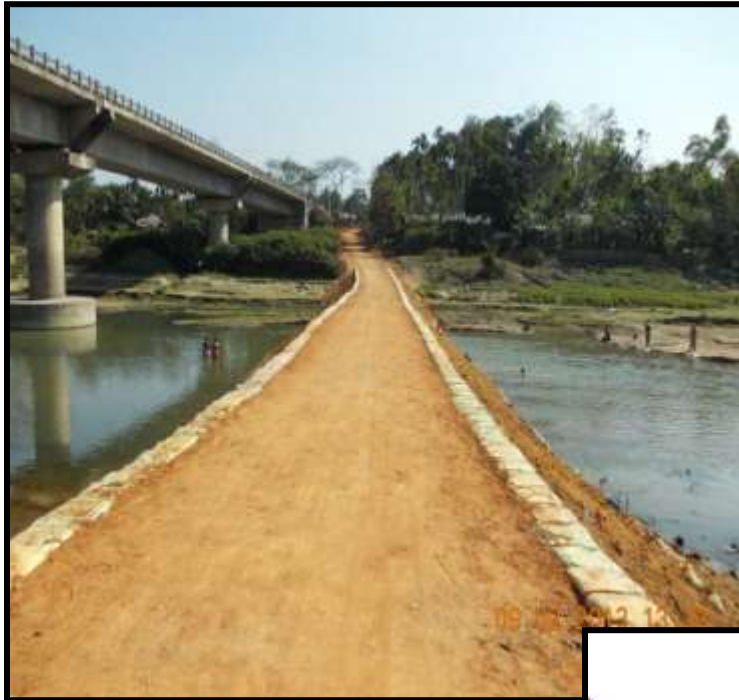
Bypass constructed at Manu bridge having Span of 4 x 47.5 mtr
