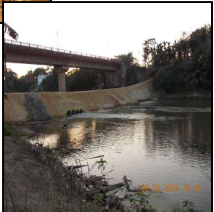
Bypass constructed at Pachertal bridge having Span of 3 x 34.5 mtr
