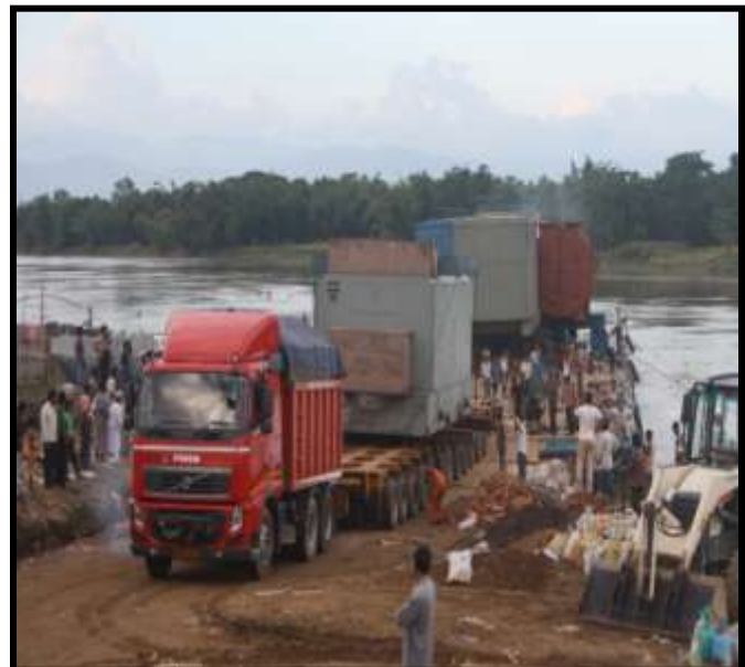
Roll off of packages through ro-ro jetty constructed by us at Karimganj on Kshuyara river
